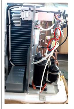
Release the three temp. sensor connectors.
